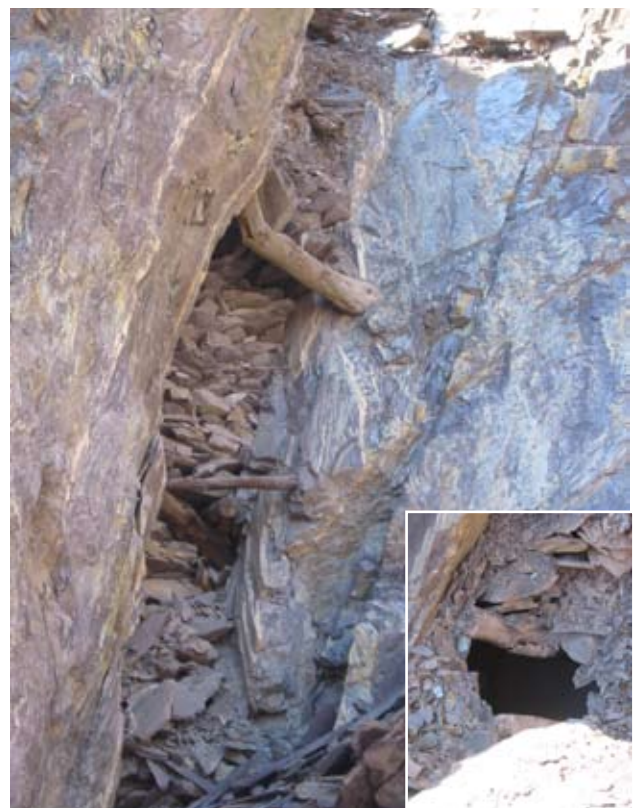
Cross-section of a former shaft, opened by Ardennes quarrying activities. The inset picture shows an opening to the lowest shaft.
